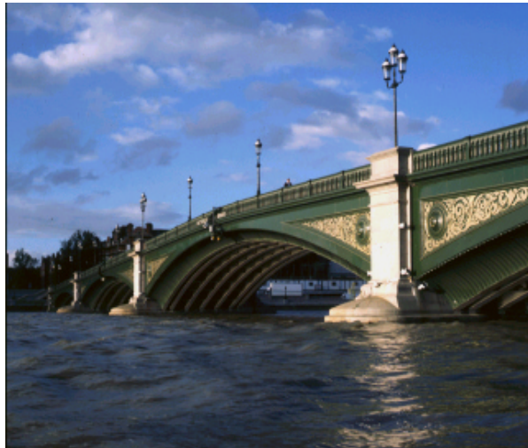
Battersea Bridge built by Sir Joseph Bazalgette in the late 1880's
